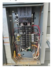
Main & Subpanels, Service & **Grounding, Main Overcurrent Device: Panel Capacity** 200 AMP
